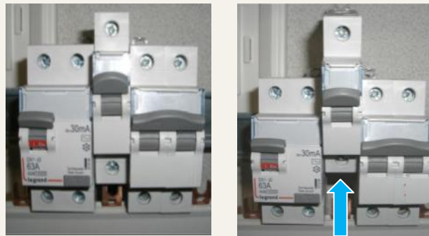
No need to unscrew the entire row
